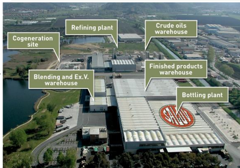
The production site – aerial photograph
